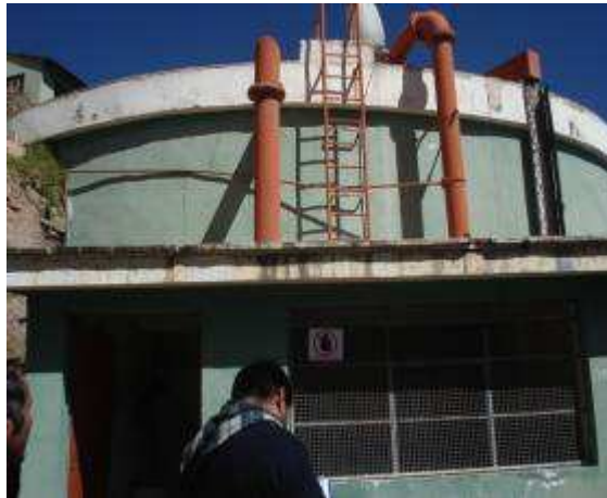
Reservorio Puerto Arturo
